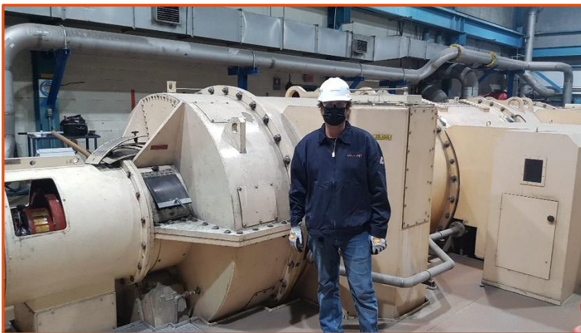
The customer's turbo generator
